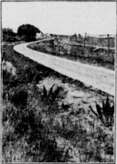
Completed Concrete Highway.
