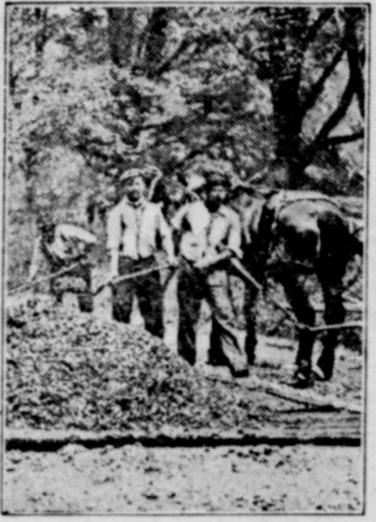
Mixing Materials for Concrete Road.
