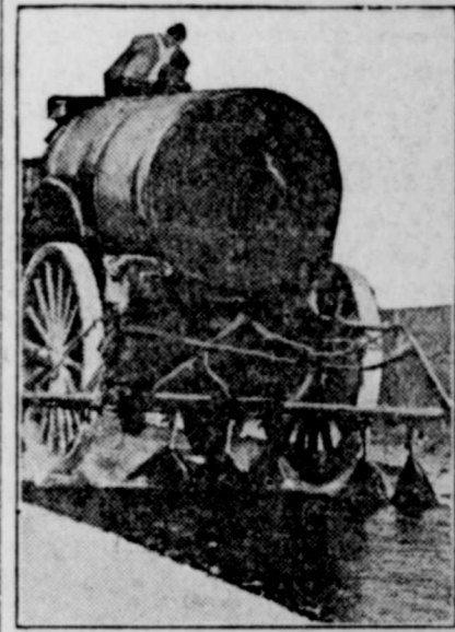
Treating the Surface of a Macadam Road With Bituminous Material.
