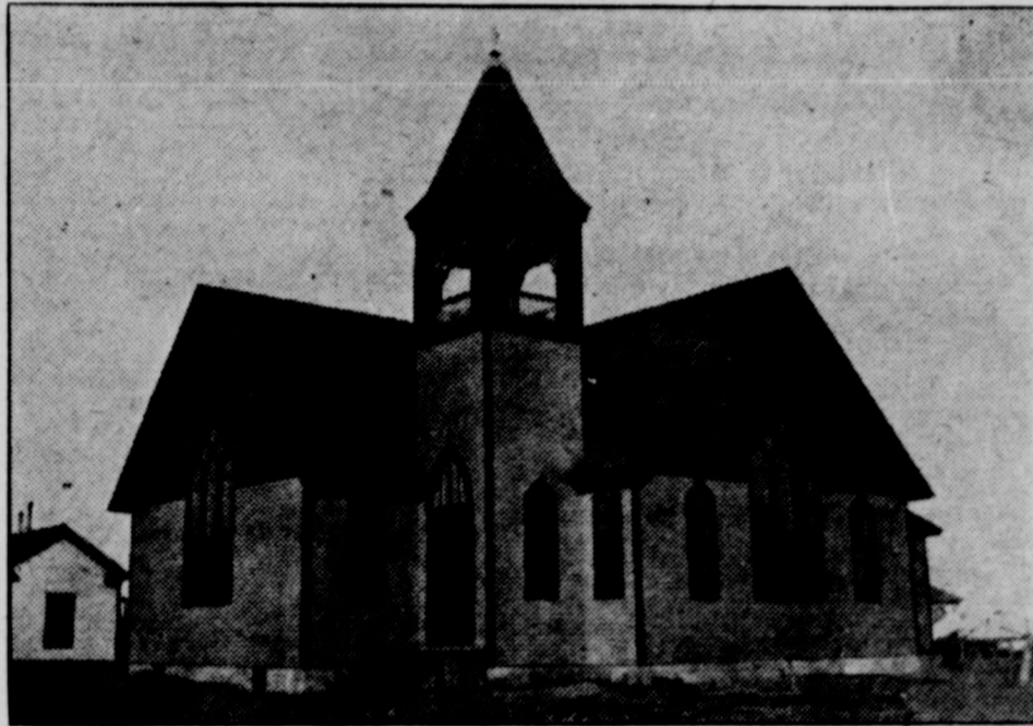
First Presbyterian Church, Artesia. Erected 1905. Cost $4,000.
