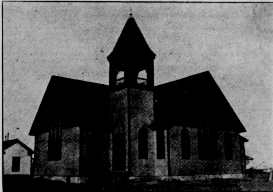
First Presbyterian Church, Artesia. Erected 1905. Cost $4,000.
