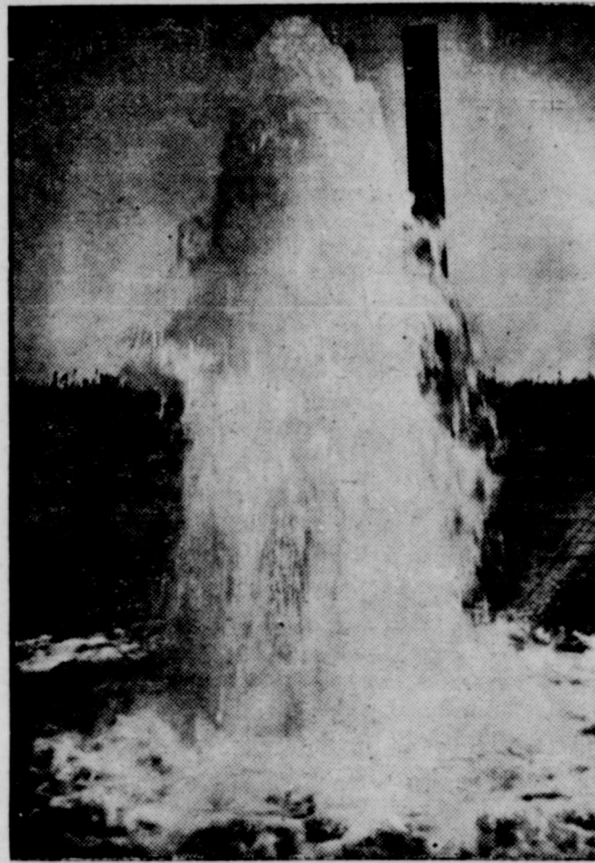
The Turknett well, two miles southeast of Artesia, probably the largest in the world, flowing 8,960 gallons per minute.—PHOTO BY TACKETT & JOHNSON.
