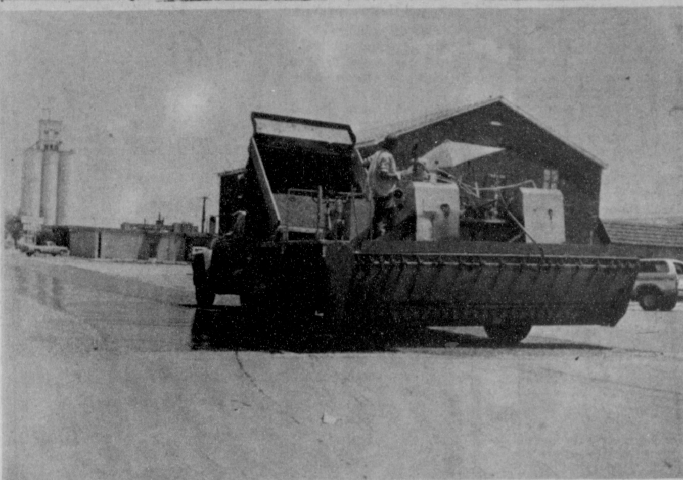
SEALCOATING OF CITY STREETS --As warm weather arrives each spring, it brings along with it a 'necessary evil.' Although drivers moan and groan about the tar flipping up on the sides of their vehicles, sealcoating of city streets is very vital and very necessary to keep streets from 'beating out potholes' in winter weather. Approximately 100 city blocks are being sealcoated in Muleshoe at this time. They are located all over the city as crews stay busy.
