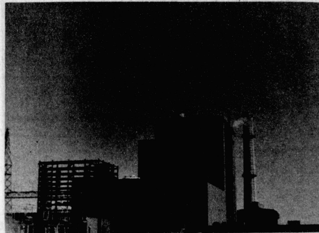
ONE DOWN AND ONE TO GO —The completed Roy Tolk Unit # 1 is seen to the right, with the structural steel on the number two unit seen in the foreground. The steel framed structure next to the finished building will house the second unit, scheduled for completion in 1985.
