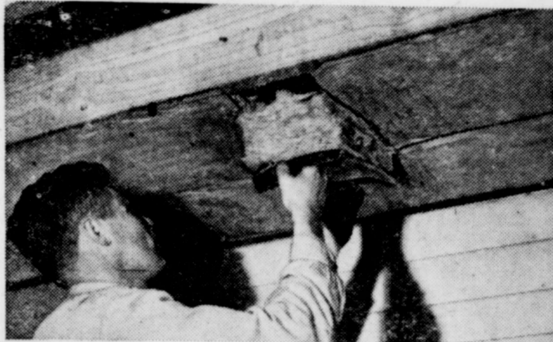
Workman carefully fits section of 6-inch mineral wool batt into place between two adjacent batts to give full, gap-free protection in the ceiling of this house being insulated for air conditioning. This goes along with the advice of home building authority Andrew C. Lang, who says: "Insist on proper installation of insulation to get full value from air conditioning."
