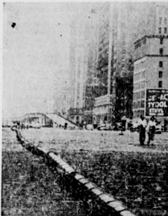
DEMONSTRATION OF PIPE in New York City which can be laid quickly over rough terrain to carry water for fire fighting, city water supply or to pump out flooded areas. This flexible-
