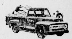
New workhorse added to the Ford line! The Ford F-350 Express with 9-ft. box. New bolted construction. Rigid tailgate. Driverized Cab! G.V.W. of 9,500 lbs. with dual rear tires. G.V.W. of 7,100 lbs. with singles.
