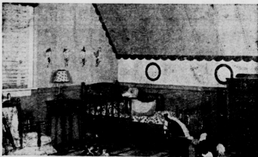
Wall board of several colors was used to turn unfinished attic into an attractive room for a child. Scalloped border was cut from the board.
