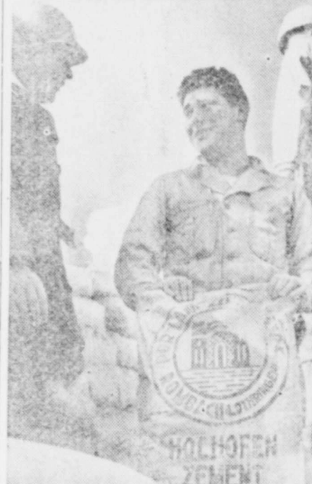
Pvt. Isidore Sack, New York, displays German cement captured in France and being used to build road to an American airport. Confiscated materials help the U. S. war effort but War Bonds pay for the vast quantity of materiel necessary for victory. U. S. Treasury Department
