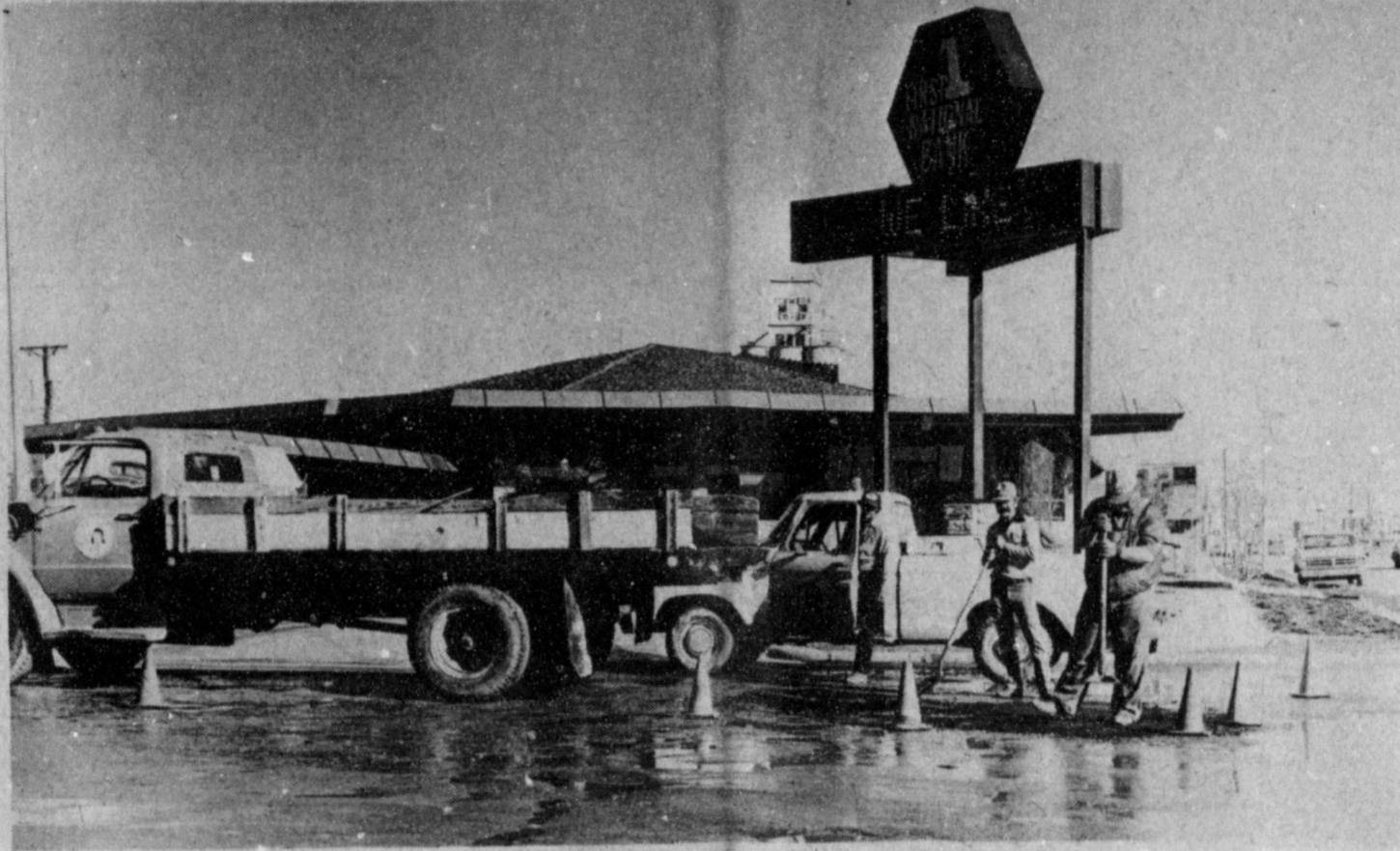
COLD, WET WEATHER BRINGS STREET WOES.... City workmen have been busy all this week repairing pot holes caused by back-to-back snowstorms that dumped around 10 inches of snow in Muleshoe each time. Many streets ended up with pot holes as traffic attempted to move on the slick, ice laden streets. At presstime, the Muleshoe city street crews had many of the streets repaired, at least until the next snow falls. After all, it won't be wintertime for nearly three weeks yet!
