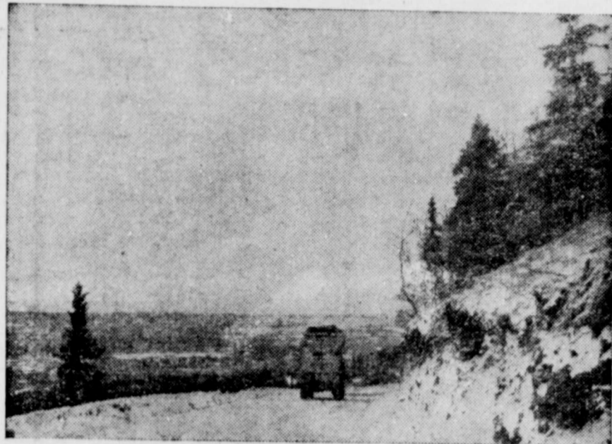
CLINTONVILLE, WIS.—More than 350 FWD trucks have helped in the almost unbelievable task of building the Alcan highway more than 1,600 miles through Canadian mountain and swamp wildernesses to open a supply road for the U. S. Army from this country to Alaska. In the picture a Four Wheel Drive truck, made here, is shown on 'suicide hill' on the Alcan highway. Later this mountainside road slid into the valley and it was necessary to reroute the highway through the valley shown in the background. The truck carries a portable camp in which U. S. Army engineers and road workers were quartered as the job moved forward. Kermit Langdok, FWD service engineer attached to the army in a technical capacity, recently returned from more than 9 months in Alaska during which his job was to keep the trucks operating.
