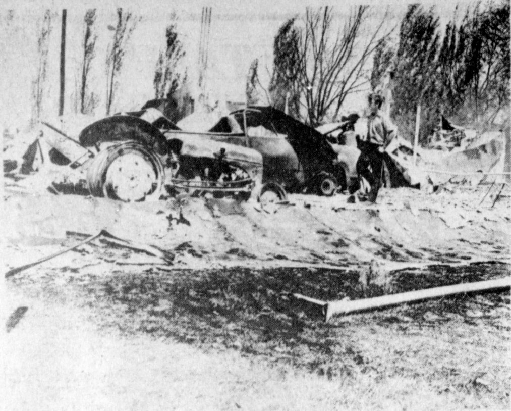
VEHICLES GUTTED IN FIRE.... Dismal remains of a tractor and plow, motorcycle and a suburban-type vehicle remained on the concrete floor of a garage at the home of Mr. and Mrs. Bob Gage following an early Saturday morning fire that totally destroyed the home, garage and contents.
