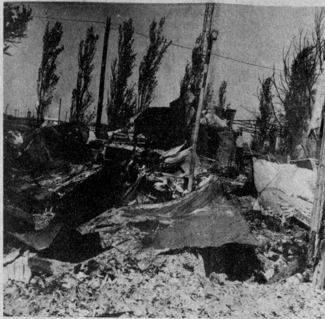
DEBRIS OF A FARM HOME.... Mr. and Mrs. Bob Gage went to Amarillo late Friday evening to help their son, Dondi, move. They were called back to their home early Saturday morning, being told their home, a suburban-type vehicle, tractor and home car had been totally destroyed by fire. They are staying temporarily at the home of her parents, Mr. and Mrs. Willis Wood.
