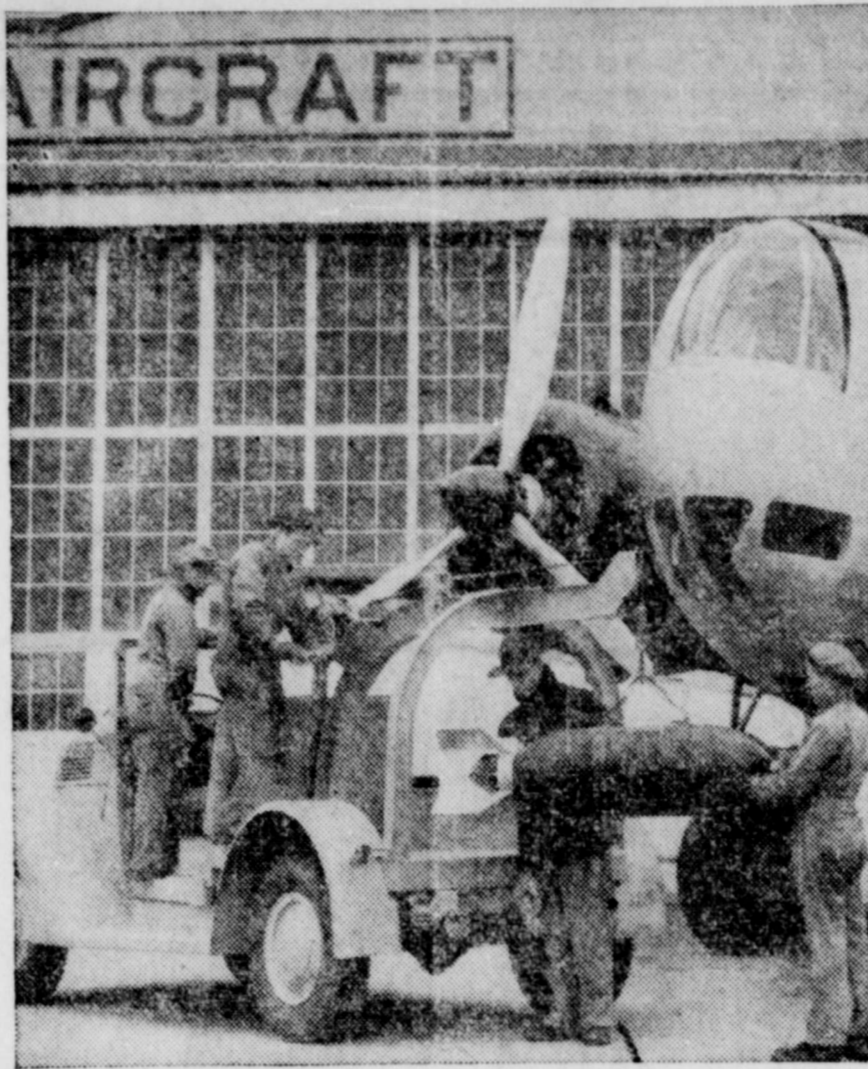
SELFRIDGE FIELD, Mich. —A familiar piece of motorized equipment around U. S. Army Air Corps bases these days is this bomb service truck, shown being demonstrated near a big bombing plane at Selfridge Field. Manufactured by the Ford Motor Company, the truck is rigged with special derrick and windlass to handle bombs weighing 600 to 1,200 pounds. The bomb in the photo is a dummy 600-pounder used for training purposes.
