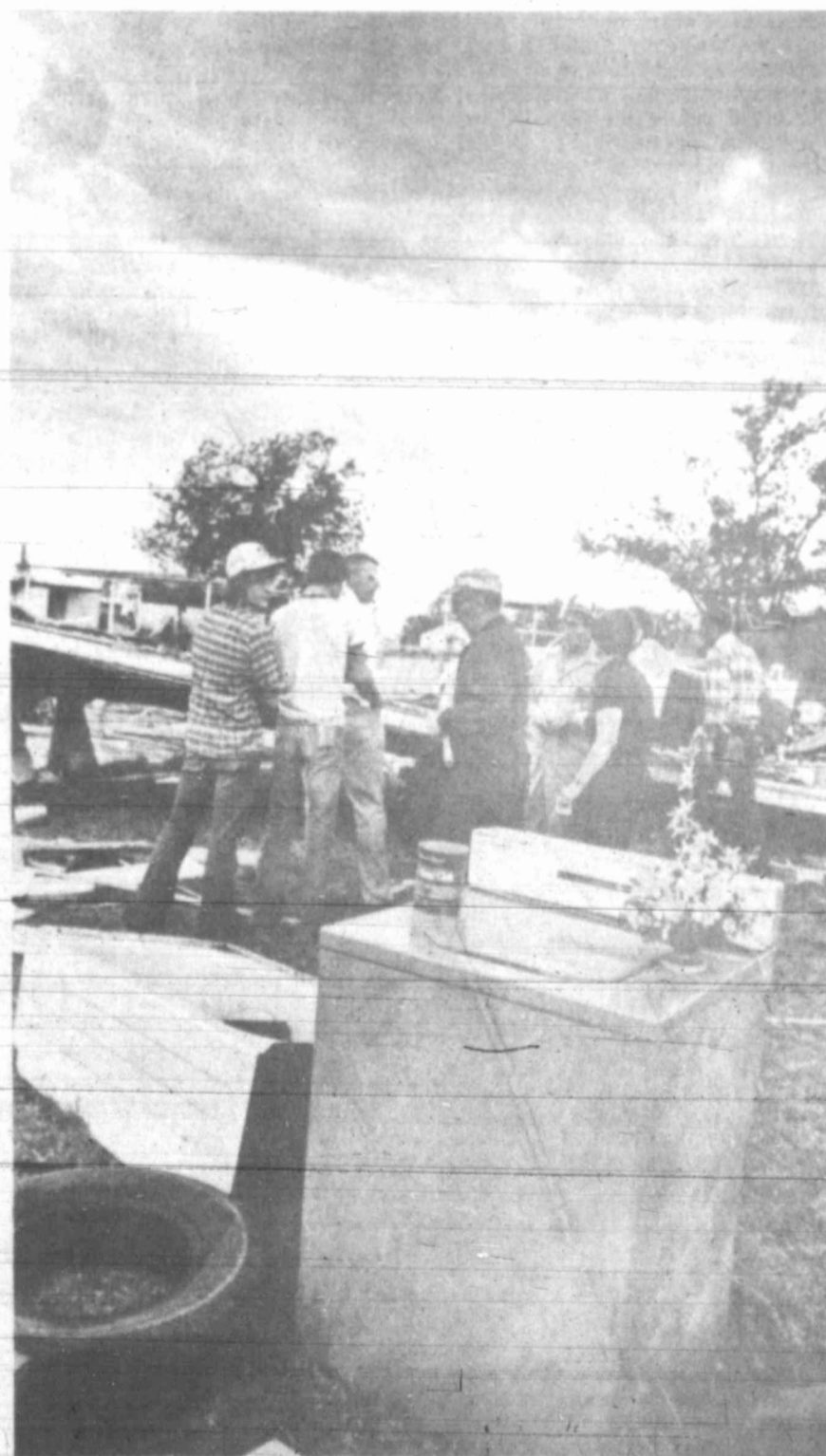
AS STORM CLOUDS LINGER, residents inspect the damage to their almost-leveled homes in Monahans. A can of coffee and a table decoration fared far better than the walls of one home and emerged unscathed.
