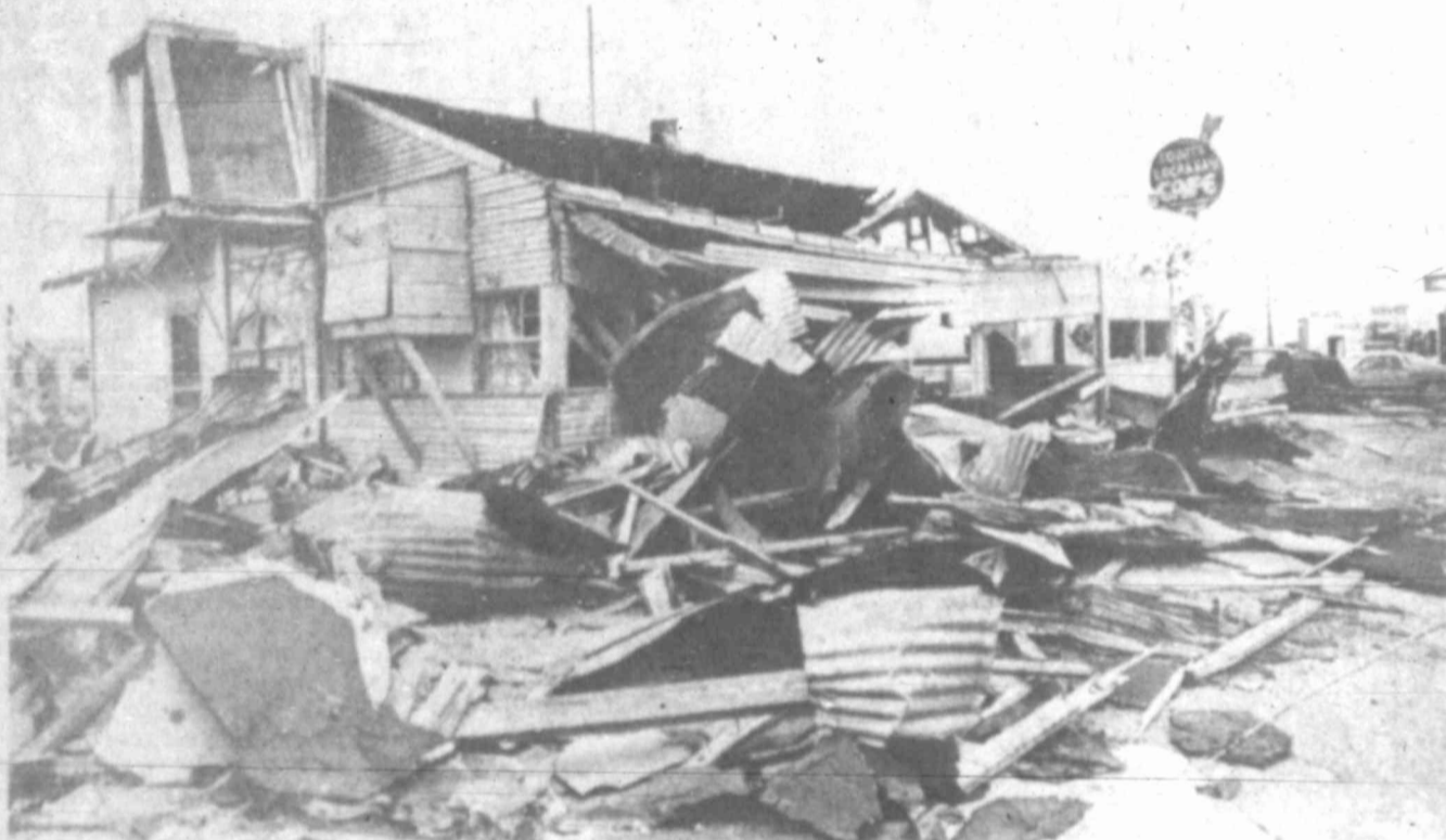
THIS CAFE on U.S. Highway 80 in Monahans is without roof and filled with debris from a tornado which struck the western part of Monahans. That
