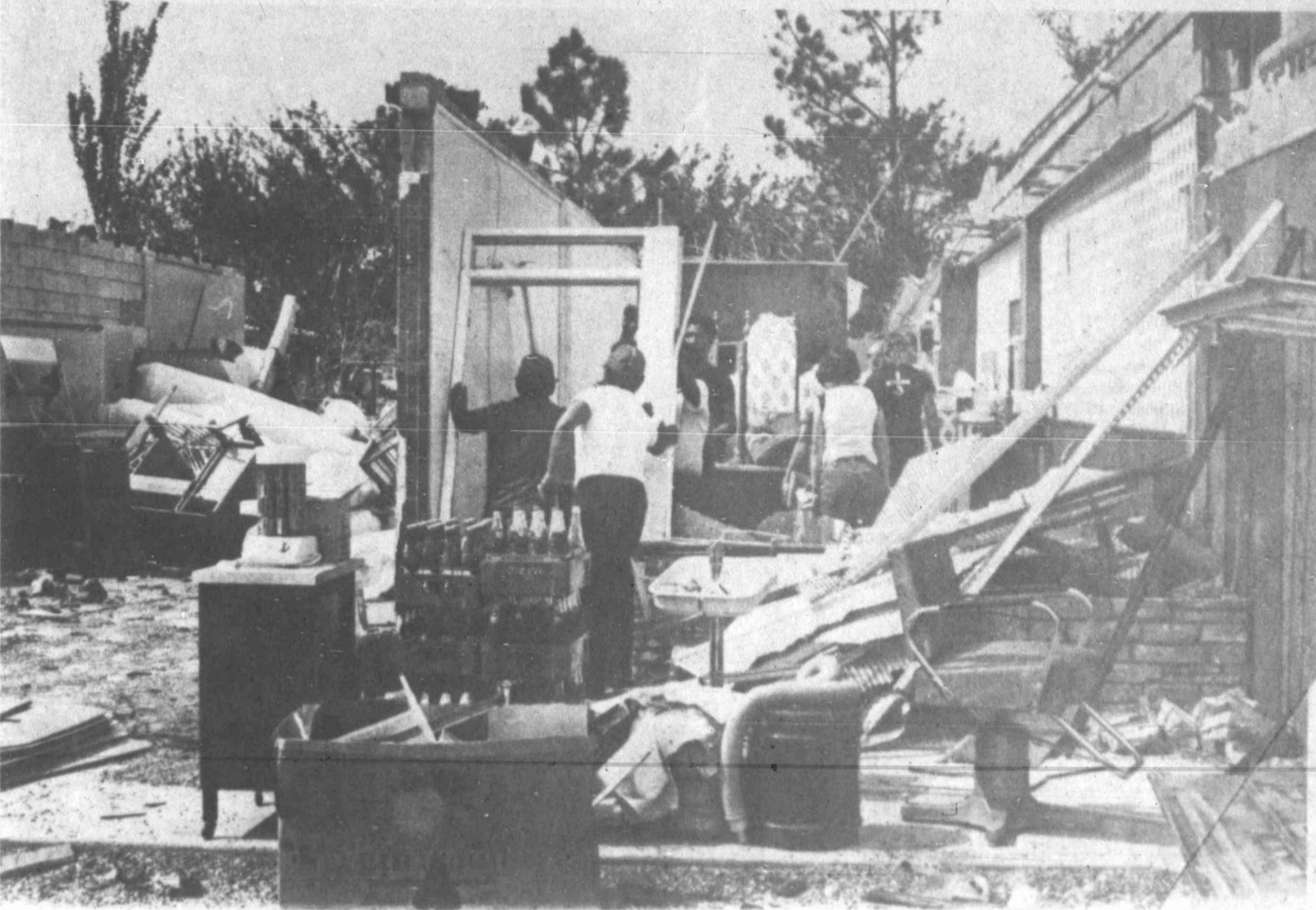
WORKERS salvage undamaged items from a barber shop which was largely reduced to rubble by Tuesday's tornado in Monahans.
