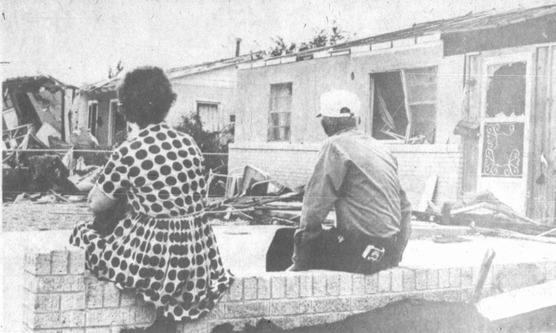
A MONAHANS COUPLE sits on an undamaged brick fence outside their home, which sustained heavy damage in a tornado.
