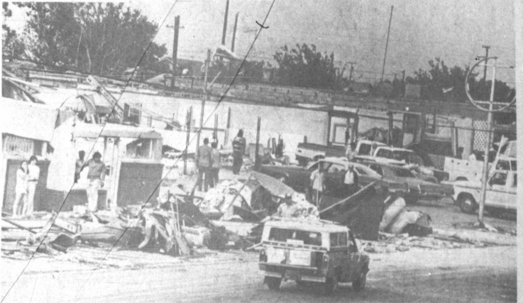
AFTER THE WINDS subsided, residents begin to assess the damage to the business district across from Ward Memorial Hospital
