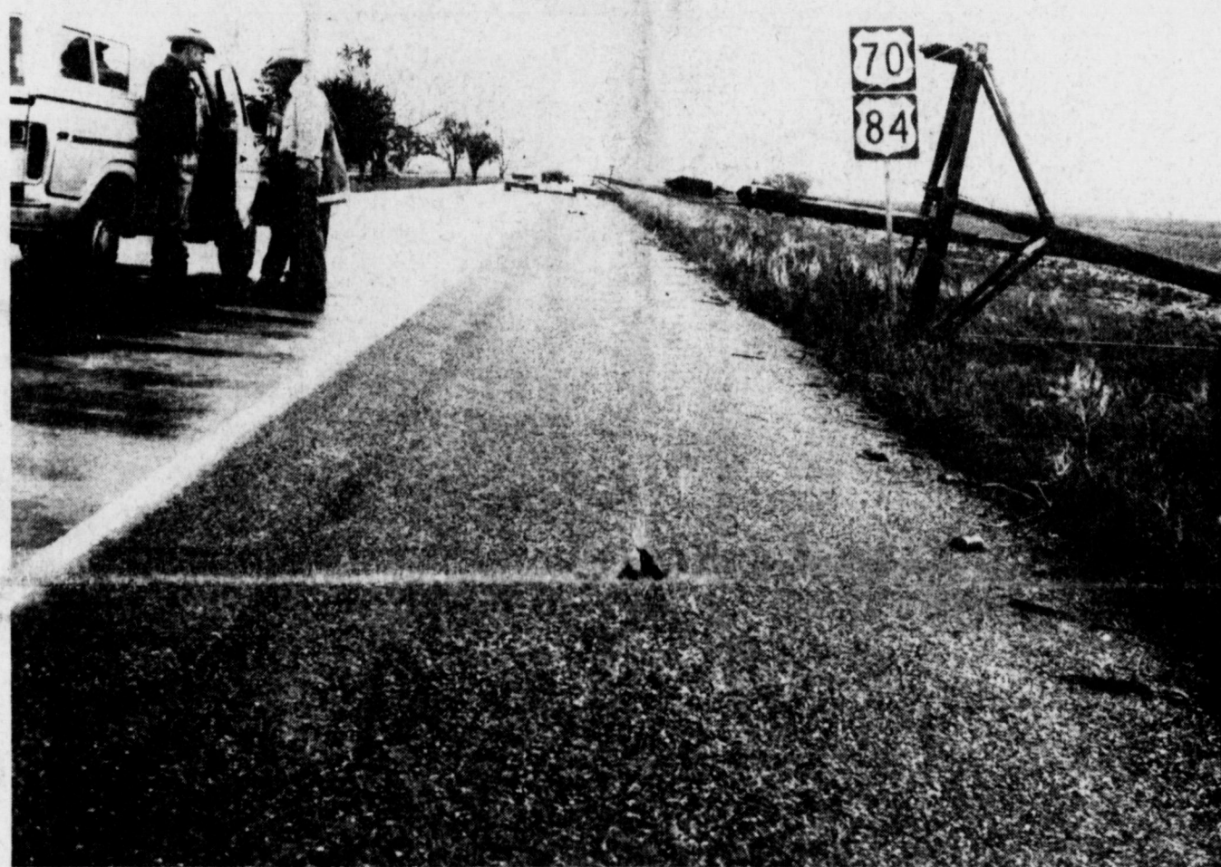
TORNADO DAMAGE IN FARMER COUNTY... Late Sunday afternoon, approximately four miles northwest of Lariat, a tornado roared across Highway 84, leaving five highline poles down, and twisting off trees in the highway median and alongside the highway. The tornado also left irrigation sprinkler pipe strewn on farms as it cut across open land. No injuries were recorded in the tornado. Here, police, fire and emergency vehicles block a portion of the highway waiting for repairs to the downed electric poles.
