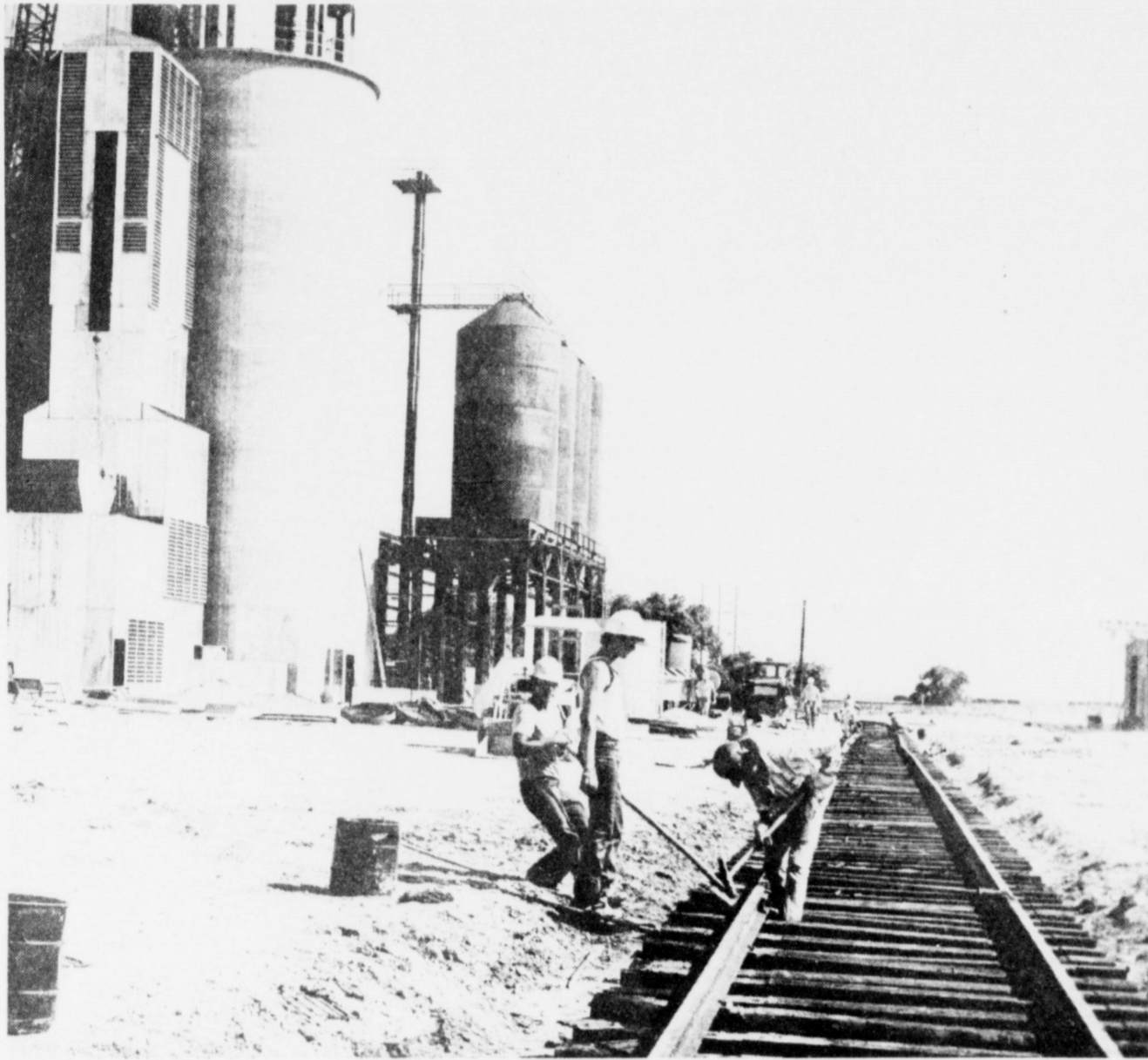
VALLEY GRAIN FACILITY COMPLETED... Initial construction of the large Valley Grain corn handling facility east of Muleshoe were completed prior to corn harvest this year. The California-based facility added a railroad spur to facilitate handling of the food corn which is held in the large tanks shown in the background. Additional construction is planned, in the future, at the location.
