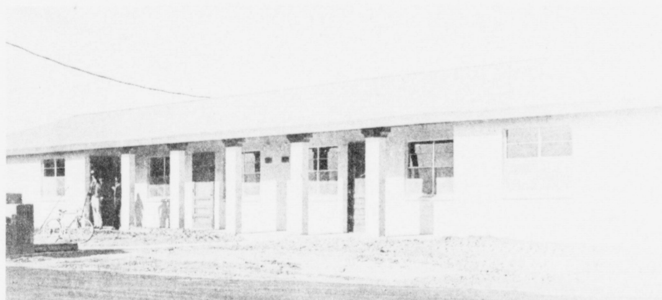
AGRICULTURE HOUSING COMPLEX OPENS... After several months of construction, the Agriculture Housing complex was completed and opened for occupancy. A total of 48 units were constructed at the site east of the city park on East Sixth Street. If necessary, the Muleshoe Housing Authority has another five acres of land adjacent to the complex for additional construction.
