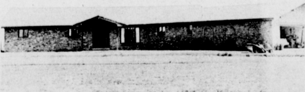
RONALD ELLIOTT HOME --Mr. and Mrs. Ronald Elliott constructed a new brick home two miles east of Clay's Corner. The Elliotts have moved into their home and landscaping has been done. The Elliott home is typical of the construction in the Lazbuddie area.
