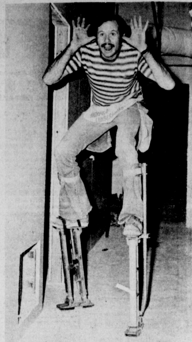
NOT ALL WORK--As this workman proves at the Bailey County Civic Center and Coliseum, it's not all work and no play. He posed for the camera Monday afternoon as he was working to install ceiling tile in the office, kitchen, meeting room complex in the building.
