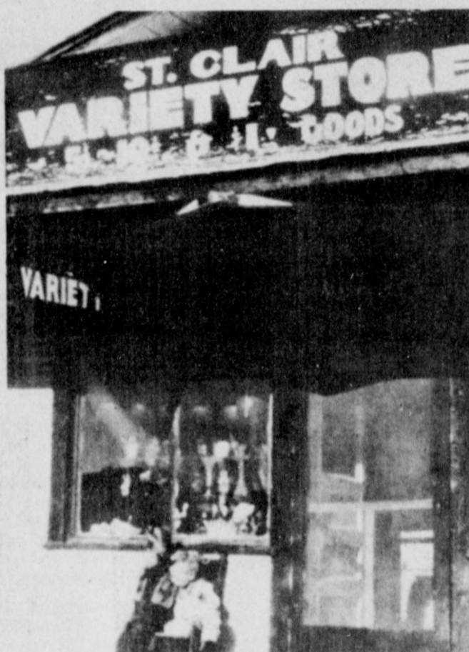
VARIETY STORE OPENED...St. Clair Variety Store opened their doors in a 25 foot store in 1930. From that time, the store has grown into its present size of 10,000 square feet. Irvin and Bill Jim St. Clair are shown in front of the original store, with living quarters in the back of the store.
