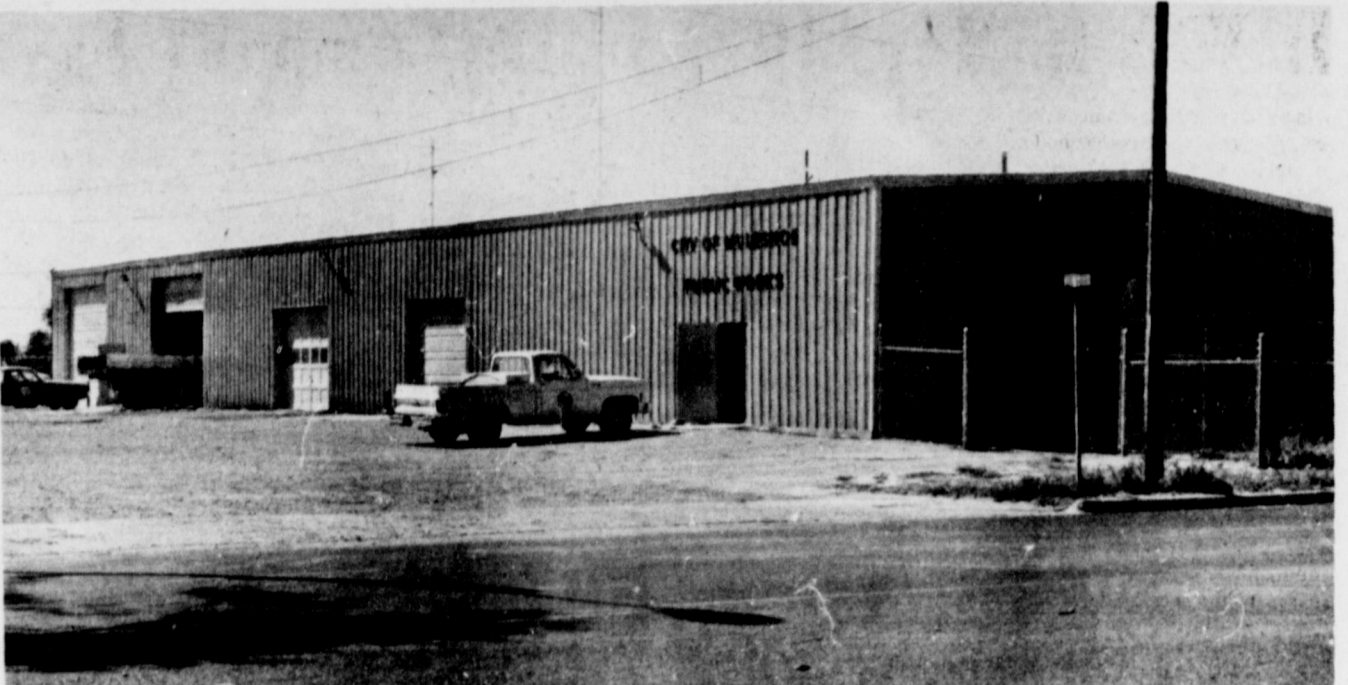
NEW CITY BARN--As Muleshoe grows, so do facilities to take care of the ever increasing needs of residents. Approximately three years ago, a new city barn was erected on the east side of Muleshoe
