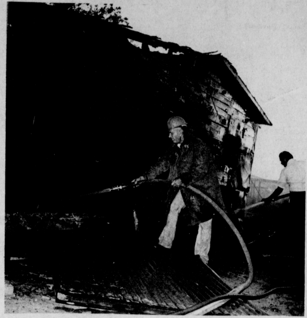
SUNDAY FIRE...Firemen Alton Carpenter, foreground and Alan Berry are shown at a fire which left much damage to the Cleve Williams home in north Muleshoe. The fire, of undetermined origin, is under investigation by the fire marshal's office. The portion shown is the garage of the unoccupied home.
