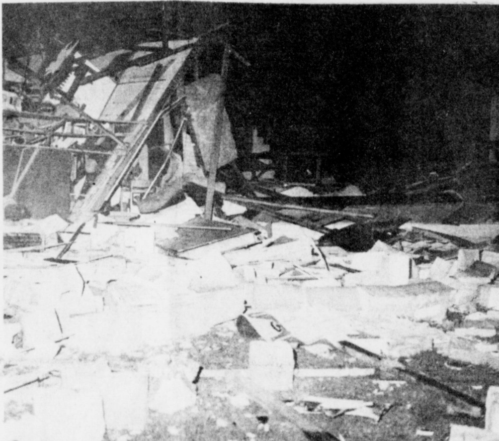
THREE WAY AG BUILDING AFTER TORNADO... Twisted steel beams and massive piles of debris mark the former Vo-Ag building at the Three Way School in southwest Bailey County following a tornado Tuesday night. Part of the steel beams from the building were in a field approximately one to one and one-half blocks from the original site of the building. For additional pictures of the tornado, see page 7 of this issue of the Muleshoe Journal.
