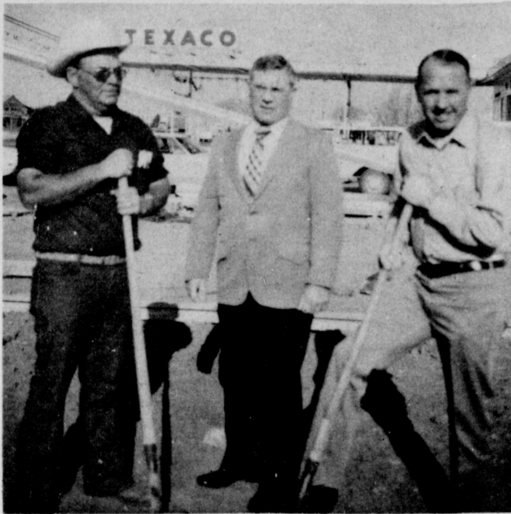
GROUNDBREAKING FOR NEW STORE . . . Lee Dunbar, left, Mayor Kenneth Henry and Howard Watson, chairman of the Muleshoe Chamber of Commerce and Agriculture Industrial Committee, turned a spade of dirt denoting the official beginning of construction of Lee's Western Wear on West American Boulevard Wednesday morning. Store opening date is set for Monday, June 27.
