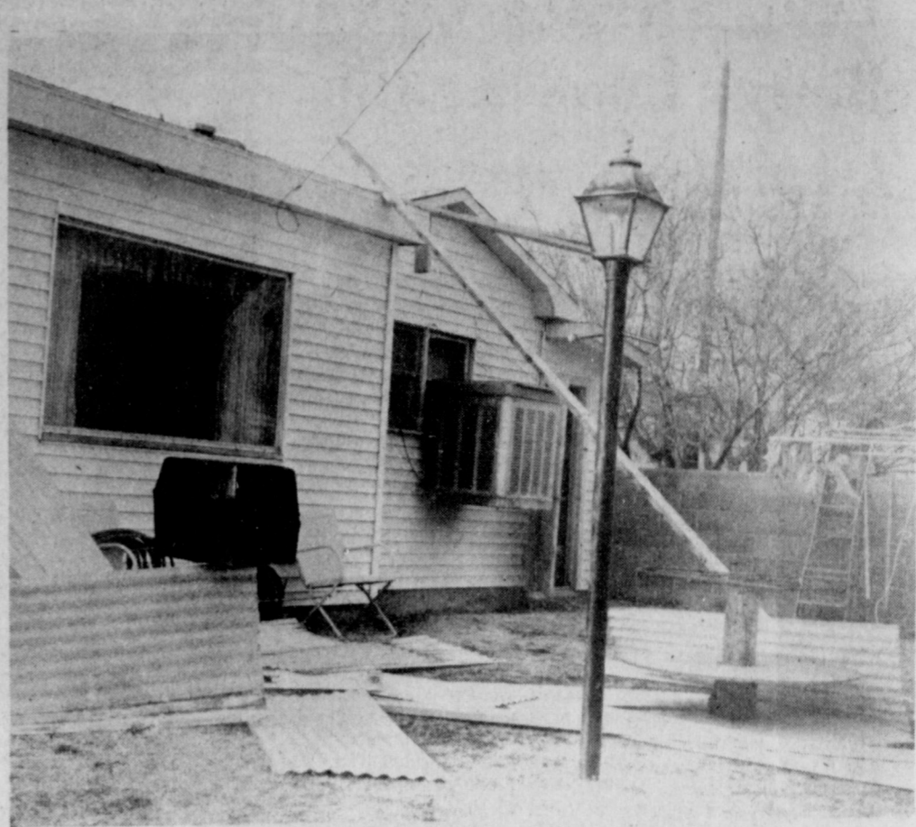
NEW CONSTRUCTION UNDERWAY? ... Now there will be new construction. The fiberglass panels and lumber were formerly a carport on the other side of the Manuel Balderas home. At least it was a carport until last Friday. High wind ripped the carport loose and dumped the debris into the backyard of the Balderas home.
