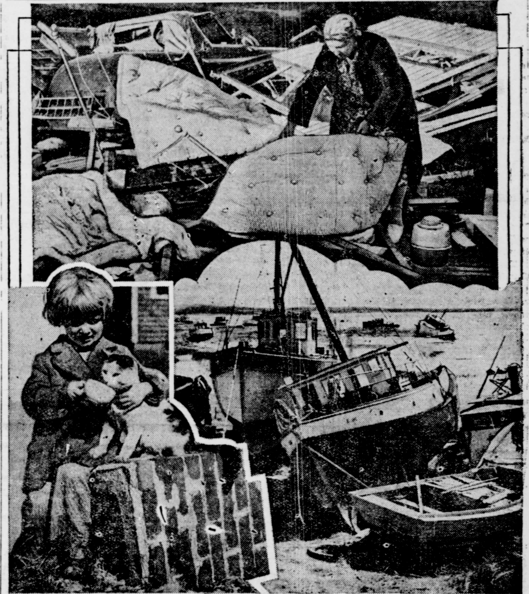
At top—Hurricane-wrecked home and motor car on Long Island; thousands were similarly destroyed. Lower right—One thousand fishing and pleasure craft were beached by tidal wave; a glimpse of Long Island coast. Lower left—Refugees from storm, seated on an overturned chimney, fed by Red Cross.
