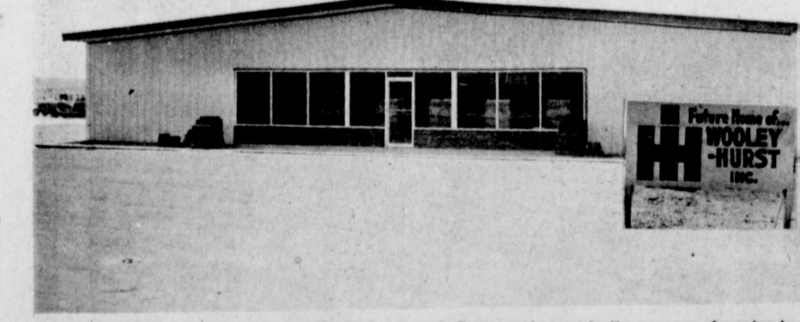
WOOLEY-HURST MOVING....Wooley-Hurst Implement Company is now in the process of moving to their new location on the Clovis Highway. The new building is located just outside the west city limits of Muleshoe. The new steel building will give Wooley-Hurst much more room and will house a shop, parts department and sales department for International-Harvester equipment.
