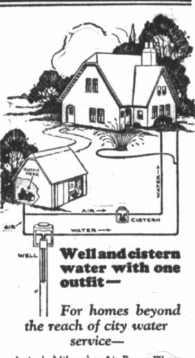
A single Milwaukee Air Power Water System gives you complete water service-hard, soft, hot and cold water at the turn of the faucet. The air com-pressor and air tank fit in a small space, a corner of the basement or garage, supplies air to operate the pumps in well and cistern. No special pump house necessary.
