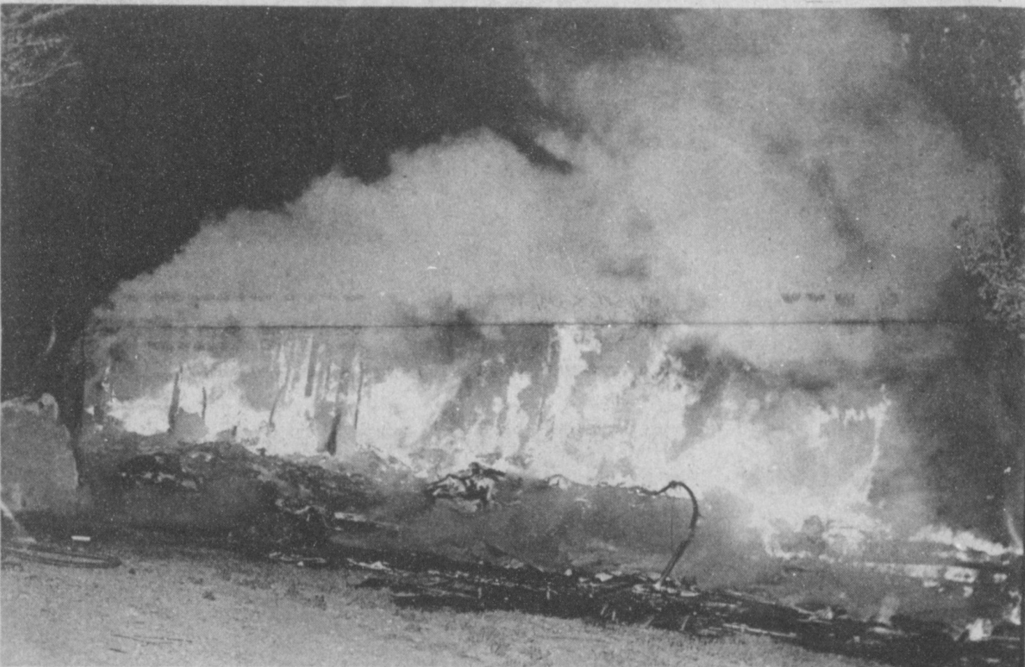
HOME RAZED BY EXPLOSION, FIRE.... Shortly after 12:30 a.m. Friday, the home of Ed Haskins at Progress was leveled by an explosion and fire. The force of the explosion blew glass, window screens and window frames into a field and across the street from the home. Haskins managed to escape from the house just before it exploded. He said he woke up and discovered the house was burning. He was not injured.
