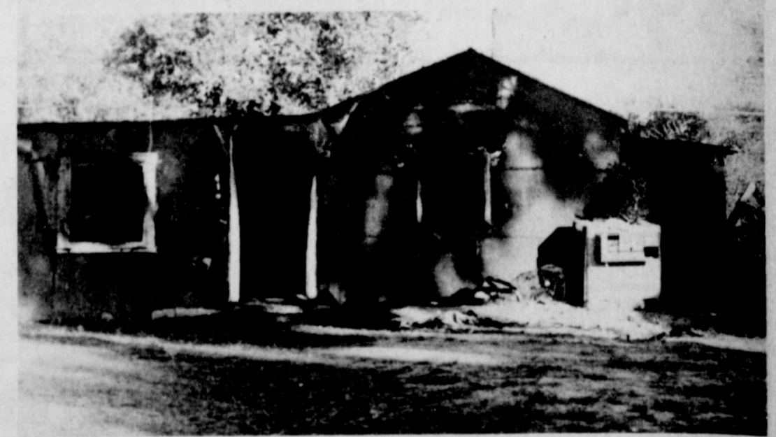
FIRE DESTROYS HOUSE . . . A fire Sunday night completely destroyed the inside of this house on East Fifth Street. Firechief Earl Ladd reports that four units of the Bailey County Volunteer Fire Department were called out at 8:30 p.m. Sunday night, but flames were going out the top of the house when fire officials arrived. The cause is still undetermined.
