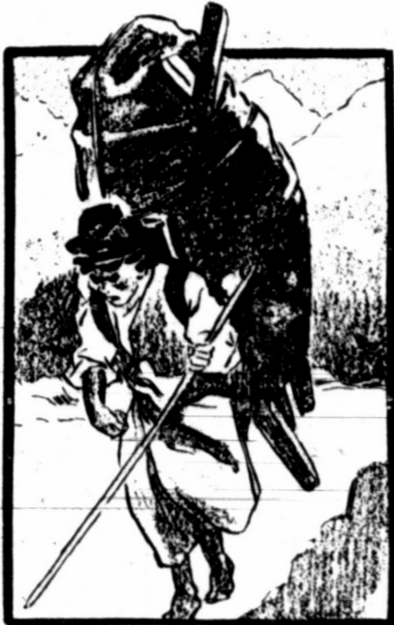
Material Carried Up.
