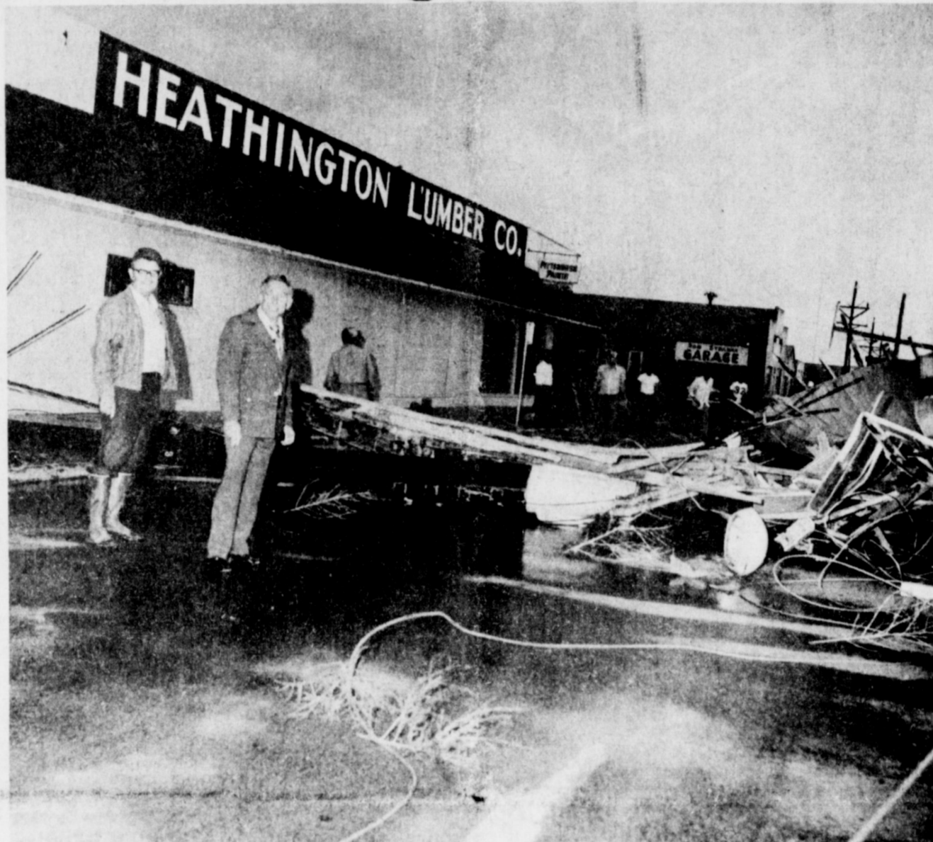
TORNADO STRIKES...Mayor Irvin St. Clair and W.E. (Pappy) Weeks are shown observing some of the damage inflicted at Heathington Lumber Company by a tornado Tuesday night. St. Clair reported that residents of Muleshoe worked together in cleaning up the streets and debris. Members of the Bailey County Civil Defense unit, local law enforcement officers, fire department members and other interested citizens were on the scene immediately to assist in the cleaning up process. The picture shows some of the debris from the building room and a street light that was twisted from the ground during the violent weather. Power lines snapped off by the twister caused the city to be without electrical power for several hours Tuesday night, but Southwestern Public Service employees worked hard at restoring power under difficult circumstances.
