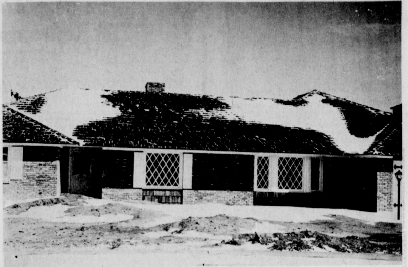
ALMOST COMPLETED...The new home of Mr. and Mrs. Bill Wooley is almost completely finished. The spacious brick home is located on Avenue H, in the Richland Hills Addition.
