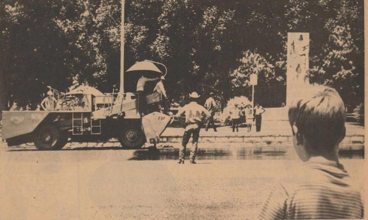
multiple units at work, simultaneously applying hot asphalt and gravel and spreading and rolling new surface, the crew
