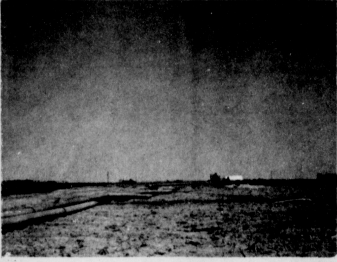
BRAIDED IRRIGATION PIPE --Shown in a braided effect is this irrigation pipe which was twisted by a tornado which moved across the country northeast of Muleshoe Friday night. The pipe is on farm land owned by W. Q. Casey.
