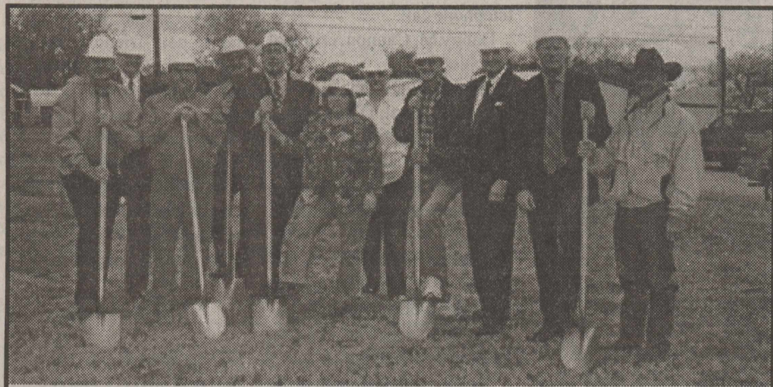
GROUND BREAKING CEREMONY — W.G. McCoy, former Bank President (from left), Glen Biggs, Bank Owner, Vernon Smith, Higginbotham's Manager, Gaylan Schroeder, Bank Director, David Estes, Bank President and Housing Initiative Board Member, Roxie Thomas, Housing Initiative Board Member, Cherry Schroeder, Don Davis, Area Housing Member and Church of Christ Pastor, Jack Griggs, Bank Owner, Steve Mack, Bank CEO and Owner, Ron Bagley, Texas Heritage Insurance Agent. (Photo courtesy of Vanda Anderson, Editor).
