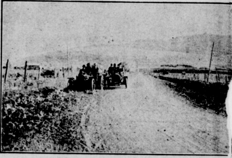
Splendid Trap Road Near LaGrand, Ore. This splendid road is near LaGrand, Oregon. It is built of Trap Rock and proven of inestimable benefit to the stretch of country. (See next page and page built. Photo supplied by the United States Office of Public Roads.)
