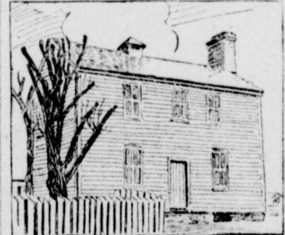
Old Lodge Building Demolished.
