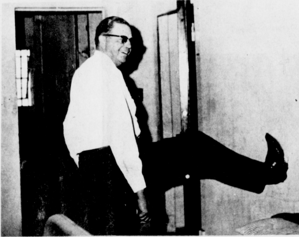
COULD BE EASY--Although Sheriff Dee Clements laughs as this picture was snapped, he demonstrates, with his boot planted in a hole already kicked in the wall inside Bailey County jail, that with some of the more experienced criminals can be so easy 'its funny' to use the term loosely. Yet it is far from funny because to keep such prisoners in custody is the responsibility of these peace officers who use the poorest of facilities to do so or carry them to another city.
