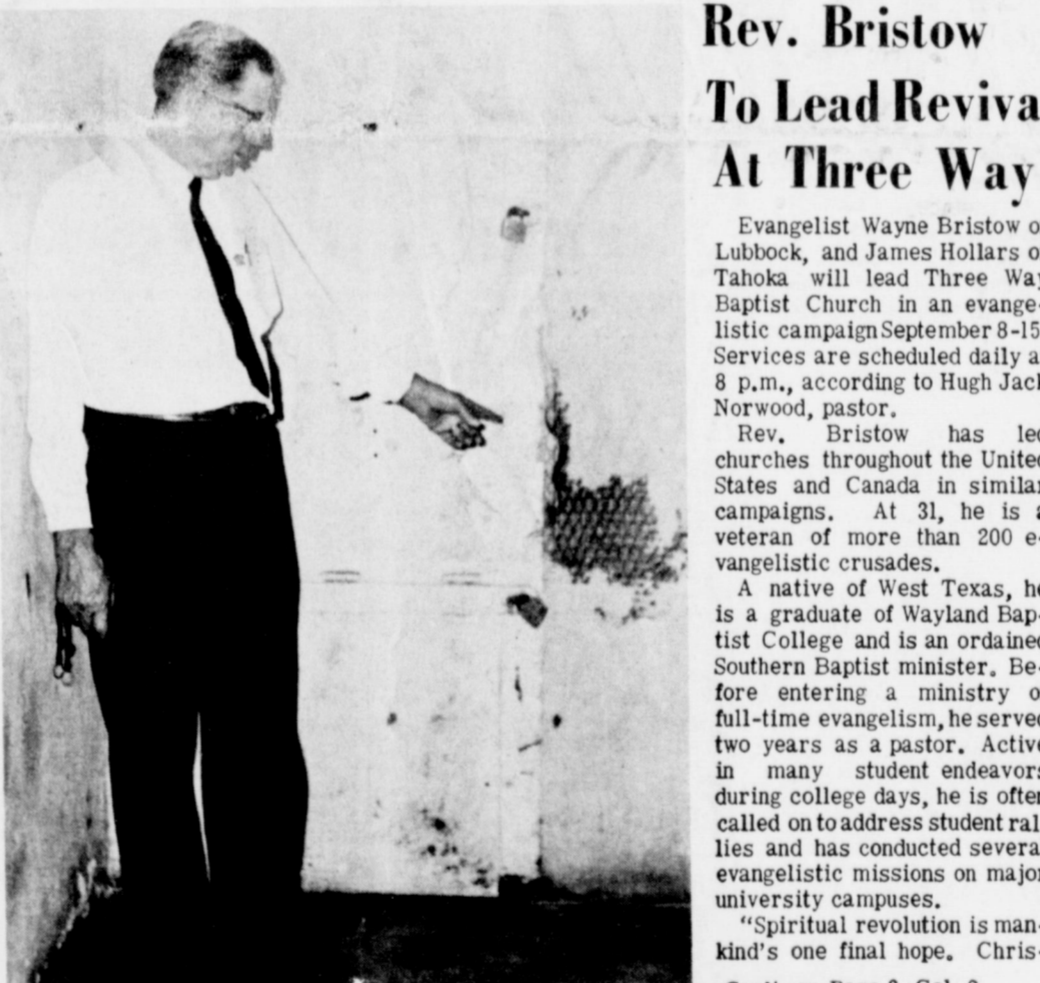
ESCAPE ROUTE--Bailey County Sheriff Dee Clements points to the spot which is the famous escape route for prisoners who had left Bailey County jail, WITHOUT PERMISSION, during years past. The lock above and below Sheriff Clements hand has been broken many times and prisoners left through a store room behind the door, by way of the roof and down over the side. The walls are also kicked in in many places inside the jail.
