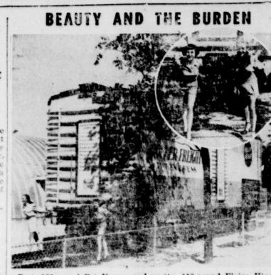
Pert, 101-pound Pat Varner and pretty, 110-pound Elaine Higgins both of Chicago, demonstrate the ease with which a 53,600-pound freight car equipped with frictionless roller bearings can be moved. The car, part of The Timken Roller Bearing Company's exhibit at the Chicago Railroad Fair, can be started with only 120 pounds of pressure, a reduction of 88 per cent in starting power, as compared to freight cars equipped with old style friction-type bearings.
