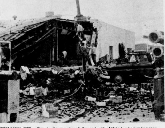
EXPLOSION SITE --- This is the remains of the east side of Muleshoe Locker Company, located on Main Street. The explosion is thought to have been from a spark from a brushtype motor which was started in the rear of the building, igniting an accumulation of gas.
