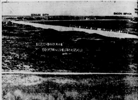
LARGEST IRRIGATION DEVELOPMENT . . . Columbia Basin project in Eastern Washington's shape. This is an artist's impression of how some of the structures in the vicinity of Coulee City will when completed. Stretching for nearly two miles across the famed Upper Grand Coulee is the South dam, which will help form a 27-mile reservoir for the million-acre irrigation development. The dam ry U. S. Highway 10-A across its top. The land will be farmed by 12,000 to 15,000 families, veteral
