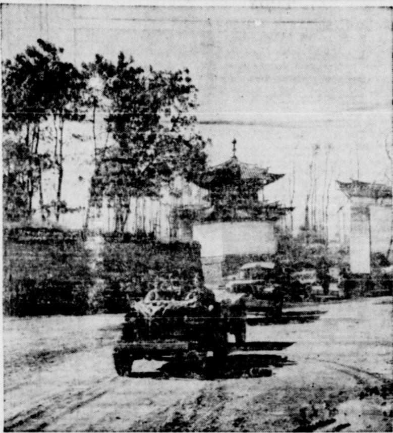
Official U. S. Signal Corps Photo. The first Service of Supply convoy over the Tengchung Cutoff, shortlink on the Stilwell Highway, leaving Tengchung on its way to Kunming terminus of this new land route to China. U. S. Army Engineers carved this shortlink out of the Burma jungles in less than three months. We can match this record at home with everyone lending full support to the Mighty Seventh War Loan Drive. From U. S. Treasury
