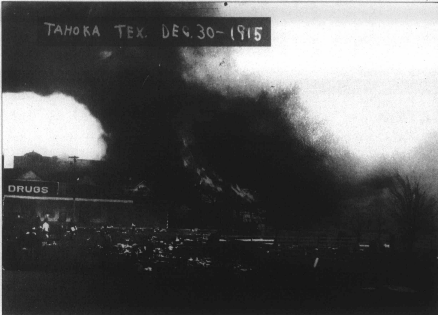
Fire of 1915 destroys Tahoka square ... "Fire wipes out one-third of Tahoka Business District" was the banner headline in the Lynn County News on Thursday, Dec. 30, 1915. Lead paragraph read: "A tiny flame of an oil heater, a blowing curtain, a blaze - where stood thirteen business houses at 9:00 a.m., by noon there lay a heap of twisted iron and smoking ashes on the north side of the public square of Tahoka. Every building on the north side of the square was almost destroyed. No one was seriously injured or burned during the blaze." (Information from pg. 118 in "Grassroots Upside Down: A History of Lynn County." The photo is on display at the Tahoka Pioneer Museum. The museum is located at 1600 Lockwood, open 10:00 a.m.-2 p.m. Fridays and Saturdays. Admission is free.
