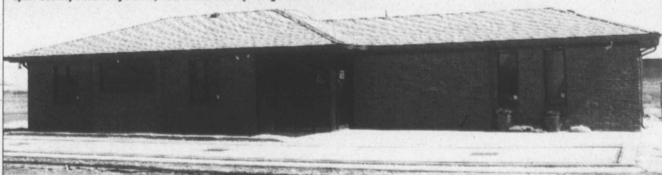
New signage will soon be erected outside this building, designating the Lynn County Justice of Peace, Pct. 1 and County Weigh Station.
