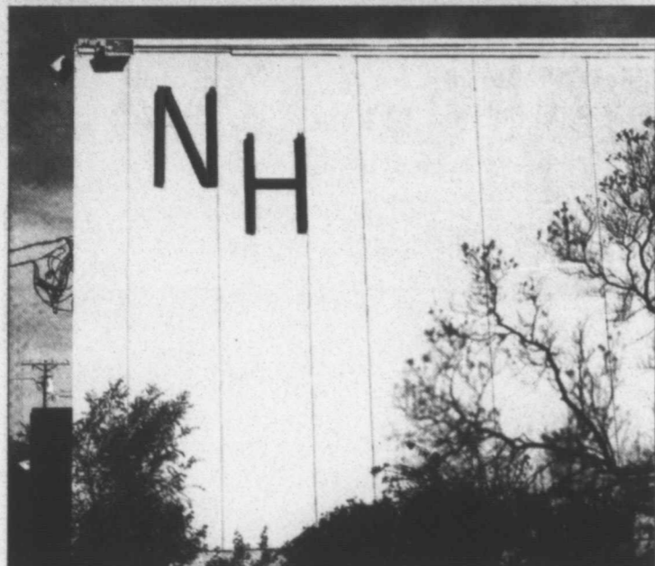
New signage ... Charles Smith, lifelong resident and former student of New Home, manufactured and donated the NH letters for the New Home ISD Gym. Mr. Smith also manufactures the Quannah Parker Trail Comanche roadside arrows. The letters were installed by Jay and Dylan Feaster, of New Home, owners of All Star Signs. "Thanks to Charles, Jay and Dylan," said a school representative.
