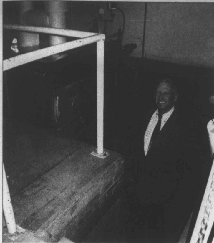
Checking it out ... Lynn County Judge Mike Braddock steps up from the sunken level in the courthouse basement where the antique boiler still sends steam coursing through the radiators of the county courthouse. Braddock says the boiler still works, although some of the large pipes to the boiler were replaced after asbestos was discovered in the basement boiler room when workers came to repair a leak recently. An asbestos removal team was hired immediately to remove it safely from the building, and new pipes were installed as well as new insulation around the machinery. (LCN PHOTO by Juanell Jones)
