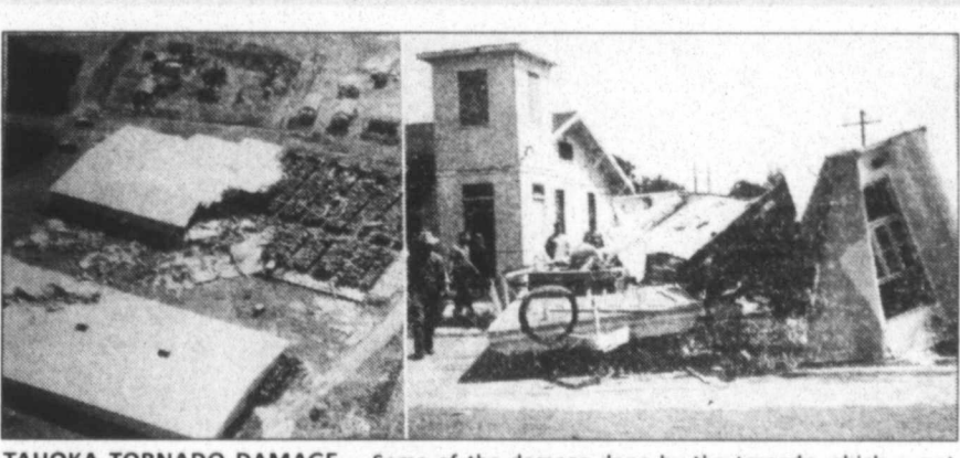
TAHOKA TORNADO DAMAGE - Some of the damage done by the tornado which swept across Tahoka and Lynn county last Friday shortly after 1:00 p.m. is shown above. At the left is one of the most severely damaged warehouses at the Tahoka Compress, while another appears to have had a bomb dropped on the roof. Center is the Nels Robinson trailer house blown across the street to the Presbyterian Church lawn. Small doll (circled) belonged to Robinson granddaughter.
