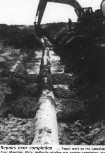
River Municipal Water Authority pipeline was nearing completion last Wednesday, according to workers on site. The 20-inch pipeline runsfrom Lake Meredith near Amarillo through Lubbock, where the water is treated, and continues south through Tahoka and O'Donnell, ending in-Lamesa. Several breaks occurred in the line 2-3 miles south of Tahoka since December, and workers have been replacing 350 feet of the pipe that runs approximately 4-ft underground on the west side of U.S. 87.
